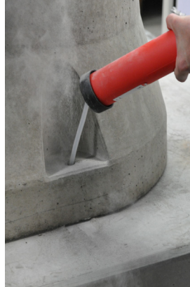
Figure 5c: Blow out the borehole
