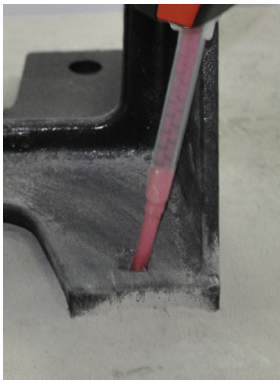
Figure 9a: Fill with composite mortar
