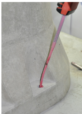
Figure 6a: Fill with mortar
