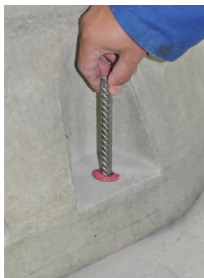
Figure 6b: Insert the reinforcement
