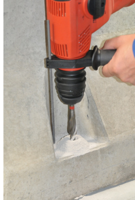
Figure 5b: Drill the fixing holes
