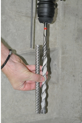
Figure 5a: Set the drill depth
