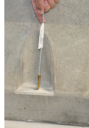
Figure 5d: Brush out borehole
